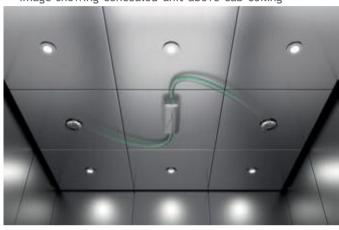
> Only inlet and outlet vents visible from within cab
